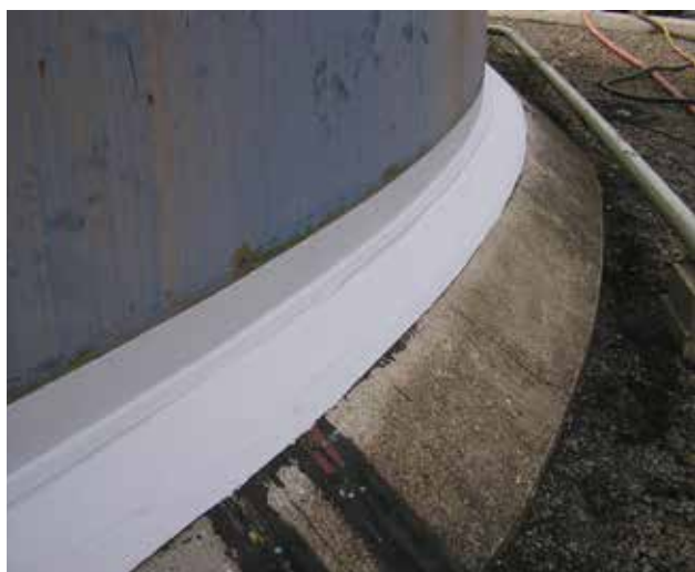
Tank base sealing
