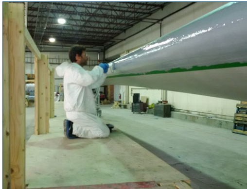
Belzona applied by roller to the Leading Edge
