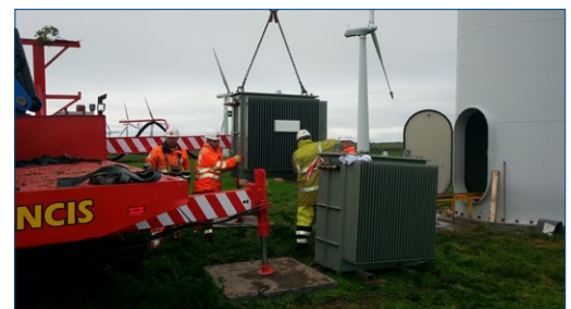
Transformer repair with Belzona 1212 VOL. XXXII, NO. 18
