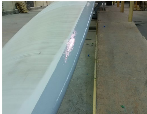
Close up of the Belzona 1341 application
