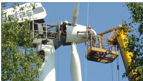
Repair within the Nacelle using Belzona 1131 (Bearing Metal) VOL. XXXII, NO. 48
