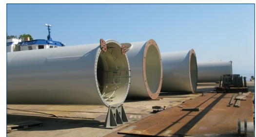
Tower repair with Belzona 1211 VOL. XXXII, NO. 33
